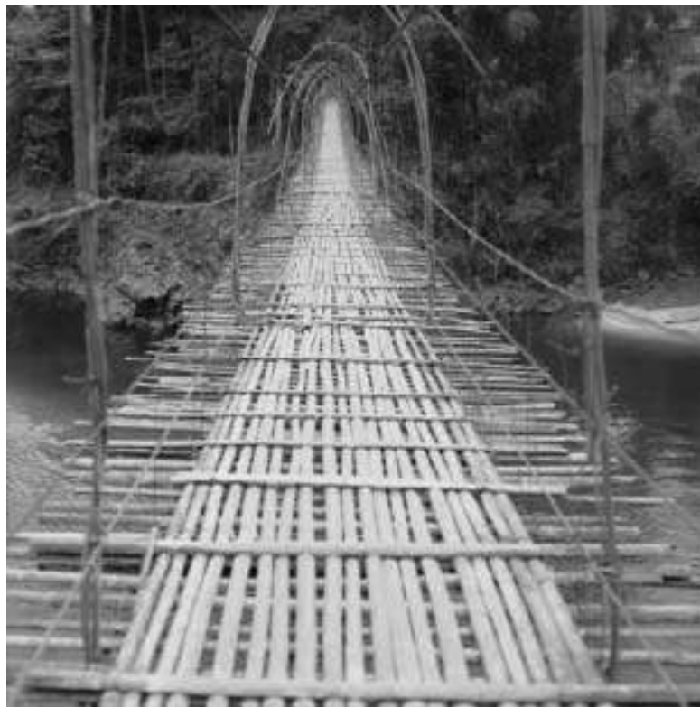
Cane-and-bamboo suspension bridge over a torrential river in Along, Arunachal Pradesh
